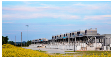
Council Bluffs Data Center
